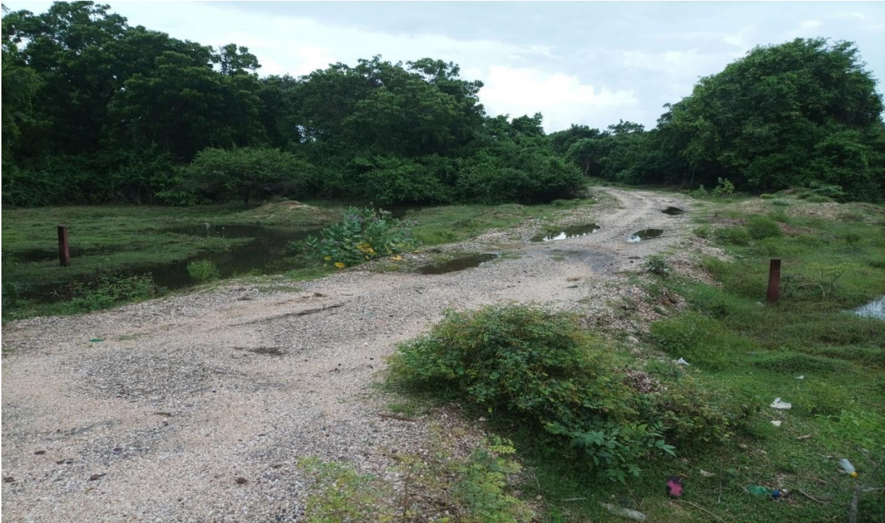
Road prepared for unauthorized transportation of sand through authority land
