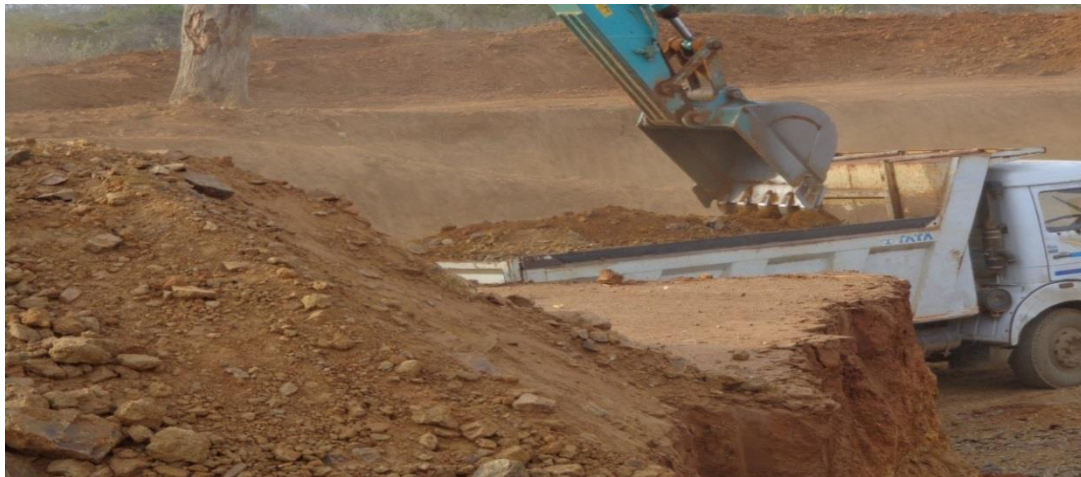
Photo 08 : A location where a license holder had carried out soil mining by contravening the conditions.
