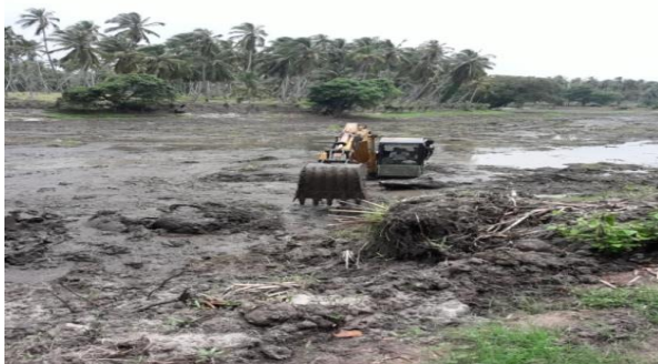
Photographs 15- Improper removal of silt in the Mahawewa, Chilaw
