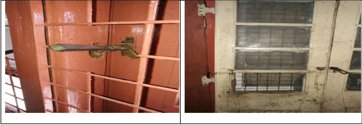
Photo 10 : Repairs carried out at the school sans compliance with the standard.
