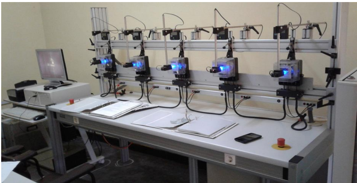
Photo 11 : The non-functional electricity meter testing facility.
