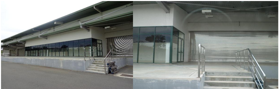
Air Cargo Buildings used for Storage of Paddy
