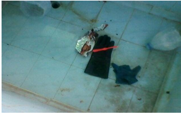
Bottom of a Water Storage Tank
