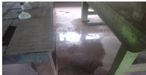
Electrical Section of the MCS
