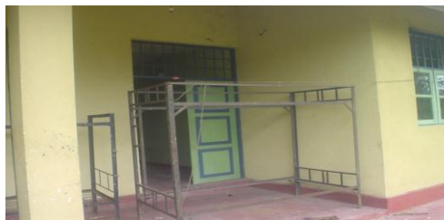
Unused Principal's Quarters
