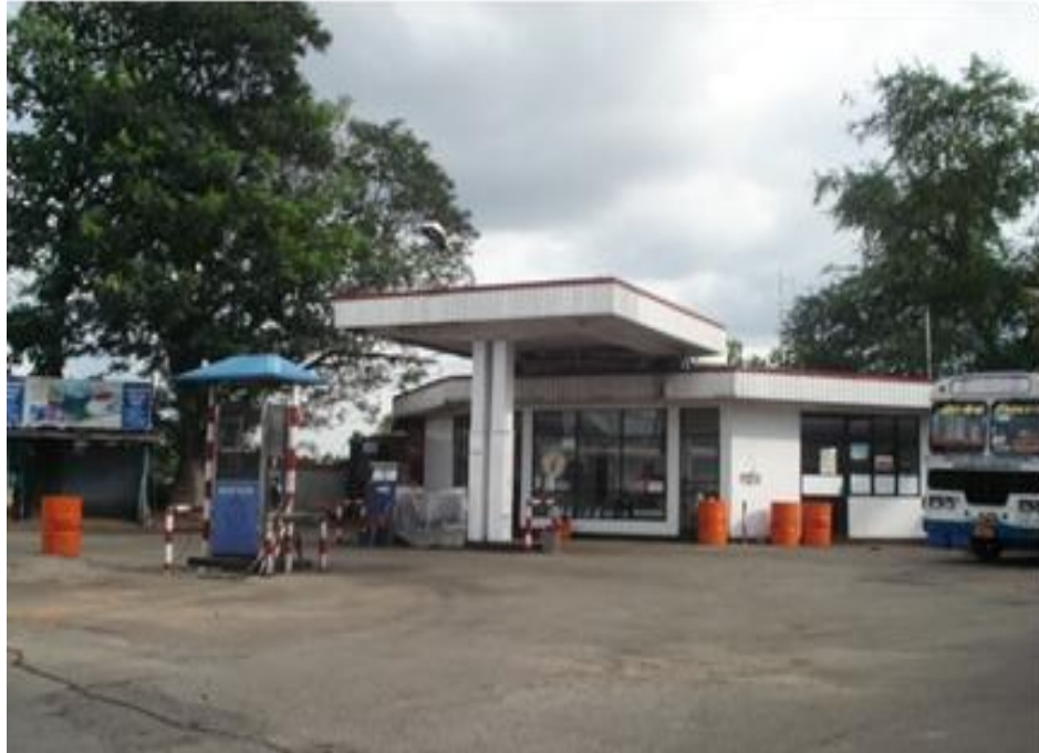
Fuel Shed at Bastian Mawatha
